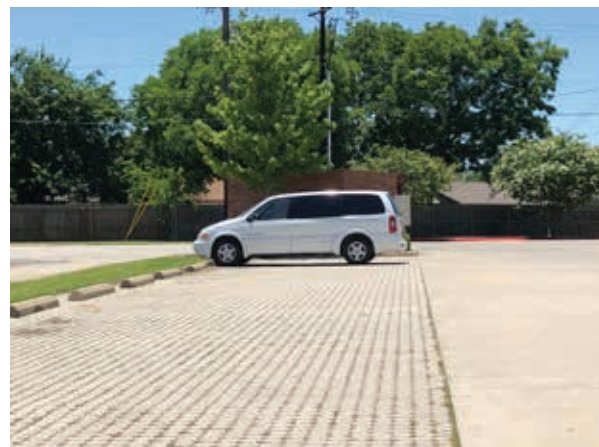
Example of Permeable Parking Surface
