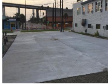
Pier/Jetty Entrance After
