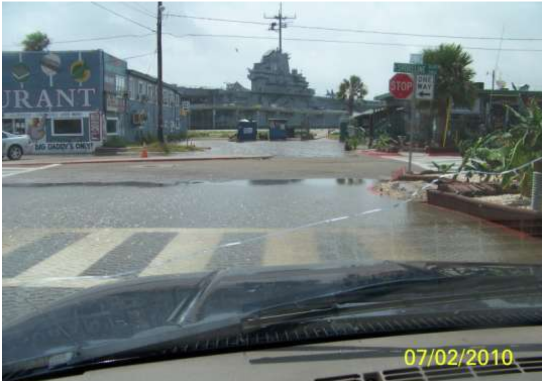
Figure 1: North Shoreline Blvd./Breakwater Ave. – East
