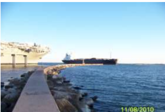
Breakwater Structure Sidewalk
