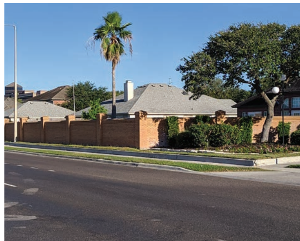
Example of High Quality Residential Fencing
