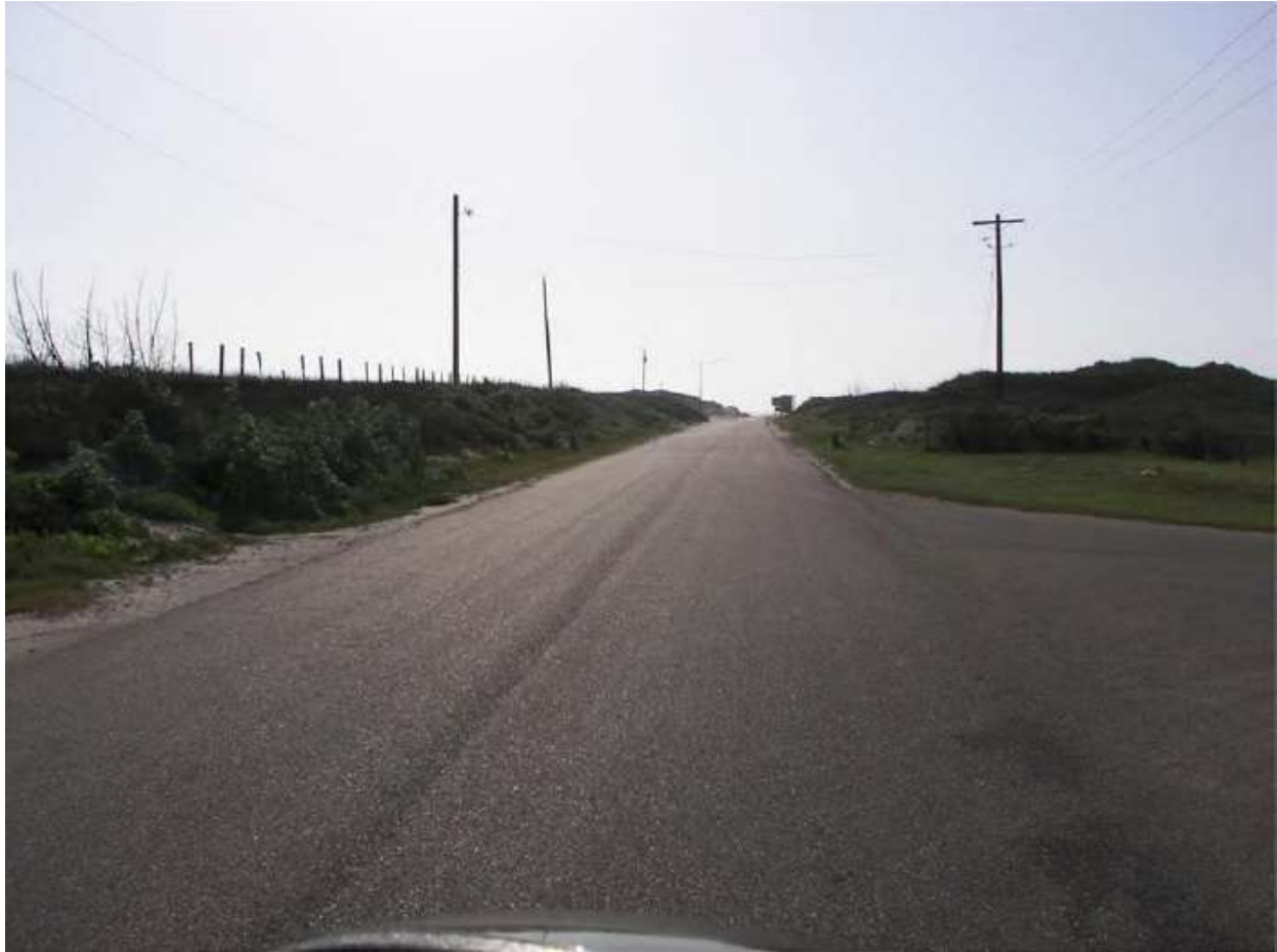
Figure 26: Beach Access Road 4, Seaward View at the Intersection of Elif Road
