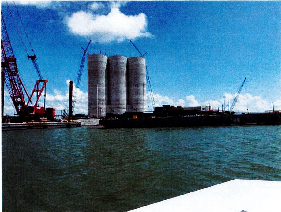
Photo 3- Photo showing northwest of proposed discharge location.
