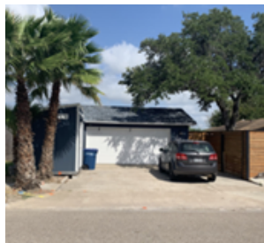
802 Oriole St. in violation for accessory structure in the front set-back.
