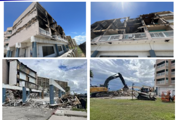
Villa Del Sol building #3 demolition in progress
