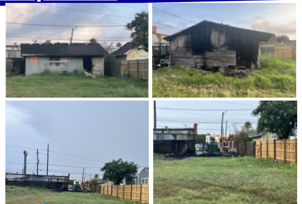
3025 David St. before & after demolition
