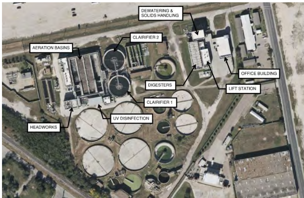
Figure 3: Broadway Wastewater Treatment Plant
