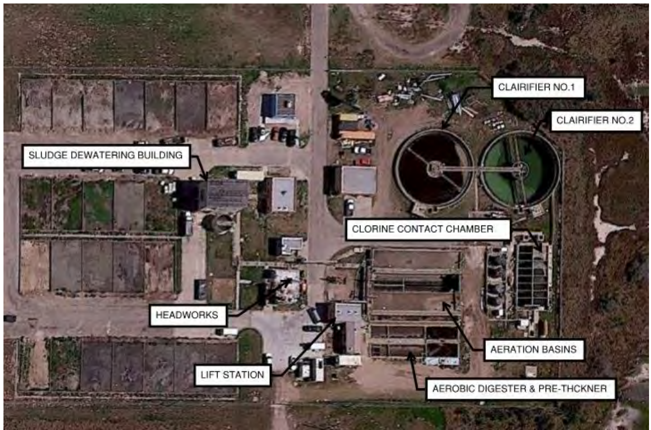
Figure 5: Laguna Madre Wastewater Treatment Plant
