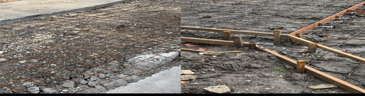
Driveways associated with commercial and residential projects that are included with the permit are not being built to city standards. Driveways should be inspected at the driveway approaches at form stage.
