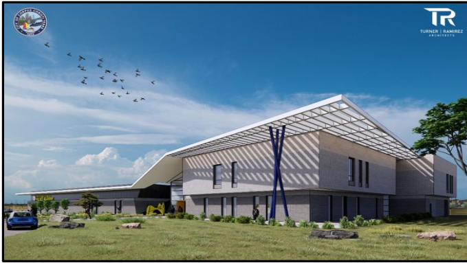
CCIA PATIO - EXTERIOR IMAGE
