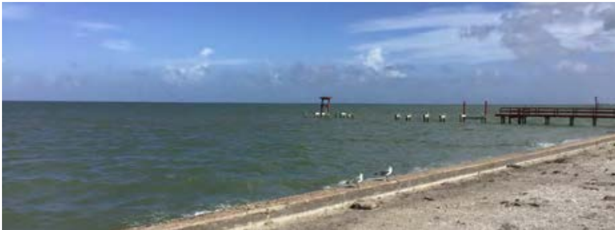
Palmetto Park seawall
