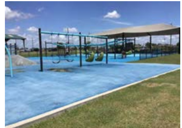
Manual Q. Salinas Park. The condition of general site facilities varies in relation to each park's classification.
