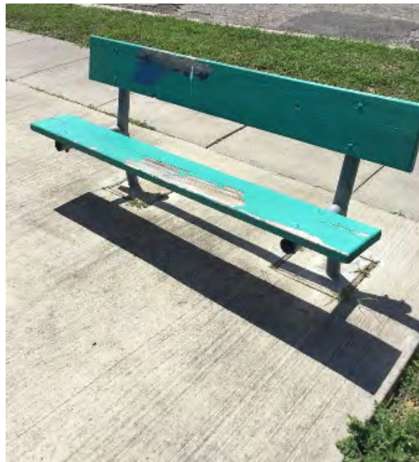
Scores for usable park amenities are negatively impacted by basic maintenance needs such as faded and chipped paint, rust, cracking mortar, etc.
