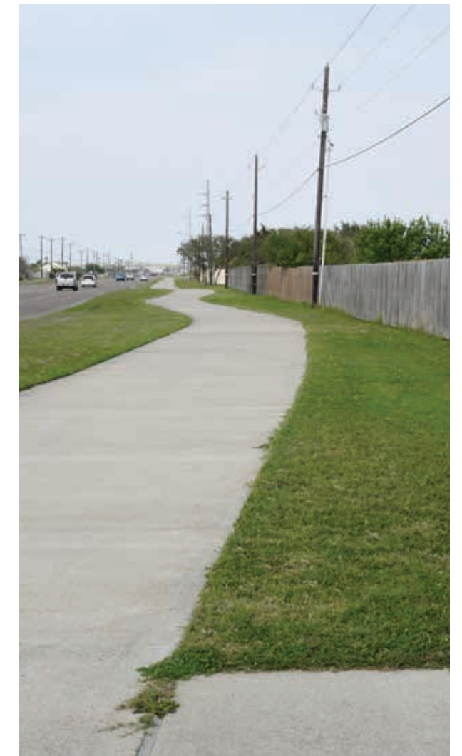
Existing Sidewalk along Flour Bluff Drive
