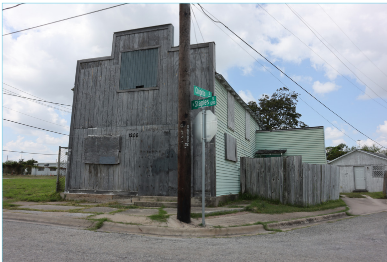
Figure 16. A vacant, boarded-up building at the corner of Chipito and Staples Streets, as it appeared in September 2020 (McDoux Preservation)
