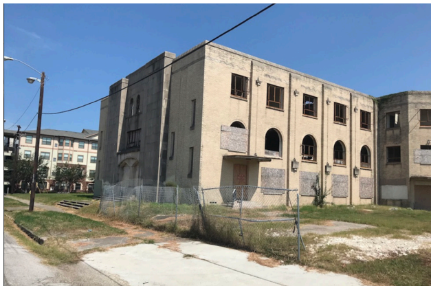
Figure 15. A vacant, boarded-up building in 2018 (Corpus Christi Business News)
