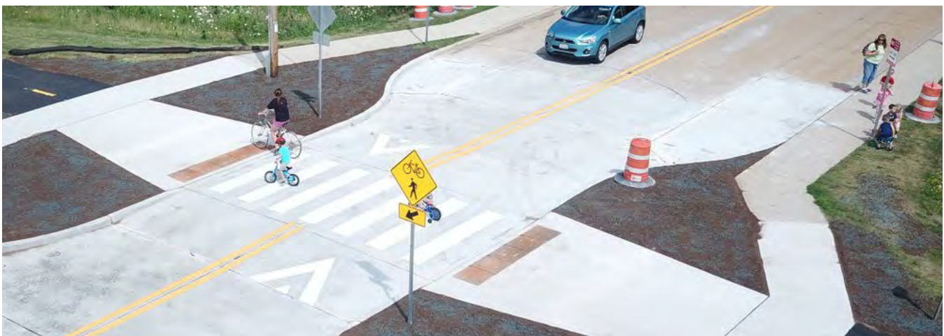
Raised, high-visibility crosswalk. Source: Appleton Department of Public Works
